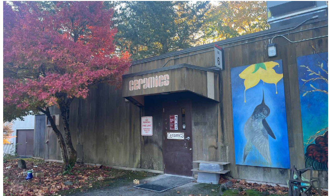
VISUAL ARTS CENTER ORIGINAL WOOD SIDING
