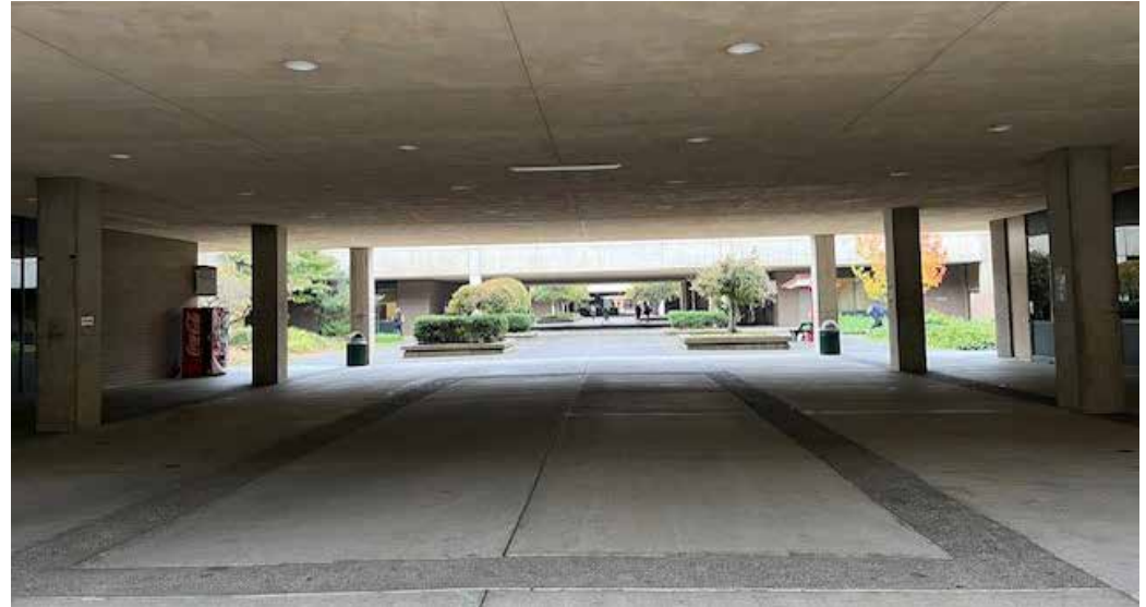
DARK UNDERPASS OUTSIDE OF CLASSROOMS
