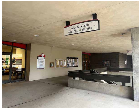
ADD COLOR AND BRANDING TO STAIRWELL
