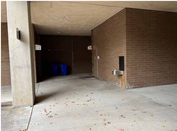
ENTRANCE TO EXISTING ELEVATOR AND TOILET ROOMS
